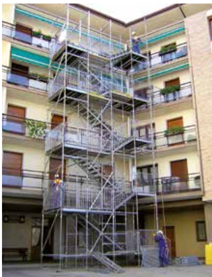
▲ Scaffolding staircase for access to flats
