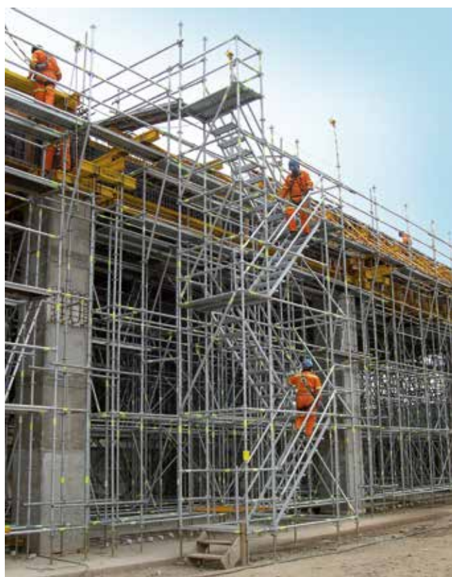
▲ Stair tower to access the formwork in the extension of the Jorge Chavez Airport, Lima, Peru
