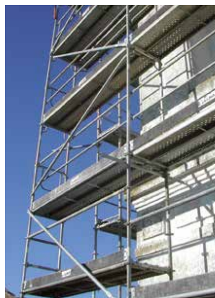
▲ BRIO Modular Scaffolding in the irregular part of the support and DORPA Frame Scaffolding in the upper part ▲
