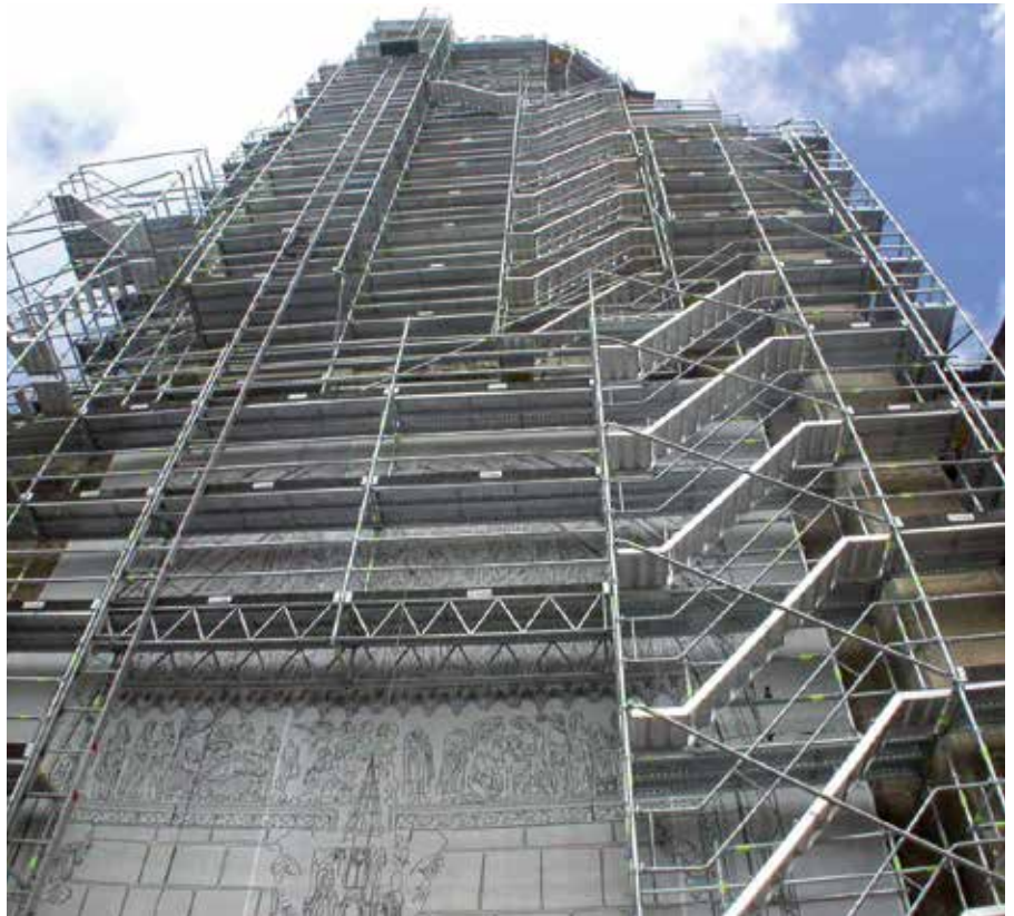
▲ Access via stairs attached to the scaffolding
