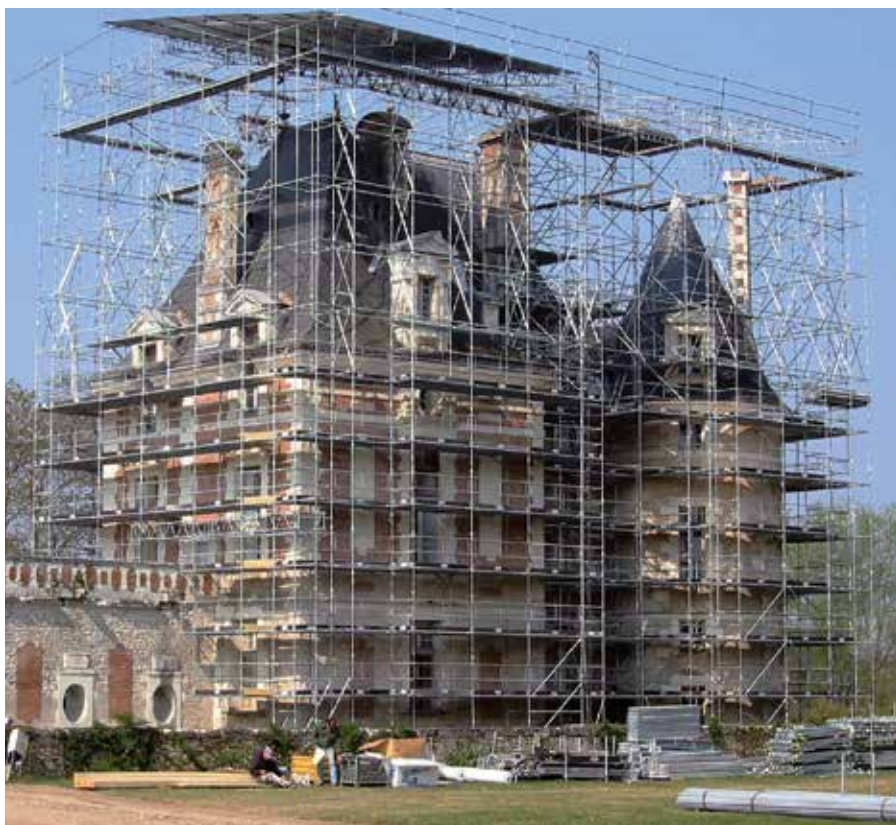
▲ Roofing at great height without possibility to tie the top level, Selles-sur-Cher Castle, France
