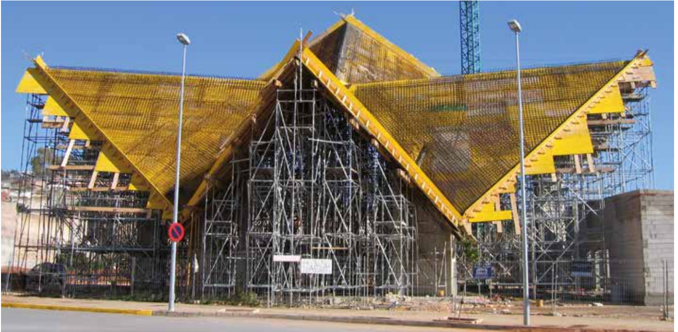
▲ BRIO Shoring System supporting the roof of the Church of the Holy Family in Alzira, Valencia, Spain
