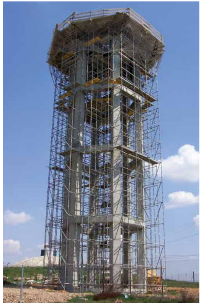
▲ Tank shoring at 24 m height
