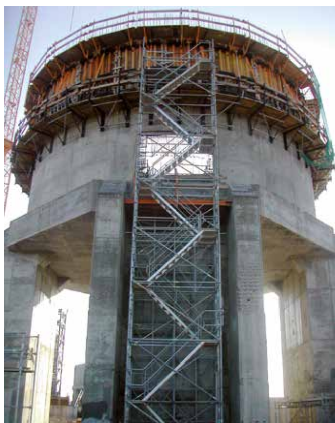
▲ Access to formwork in silo construction
