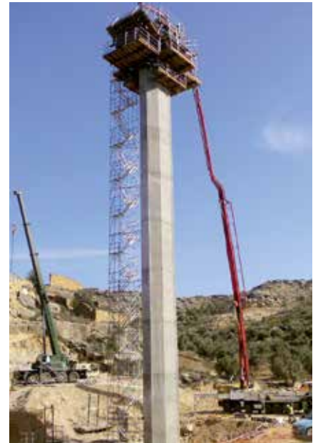
▲ Stairs to access the pier head formwork
