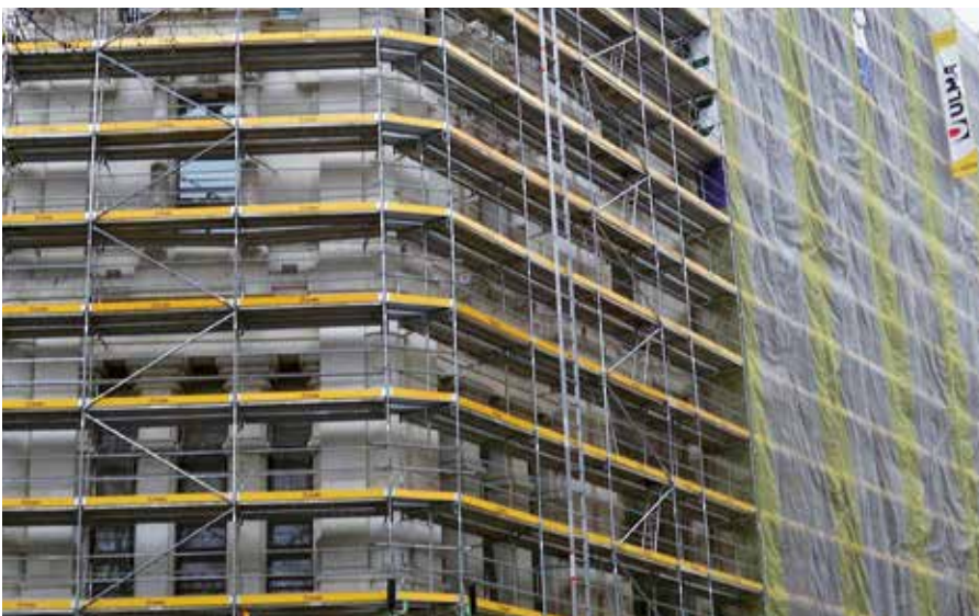
▲ Working levels protected with guardrails and toeboards
