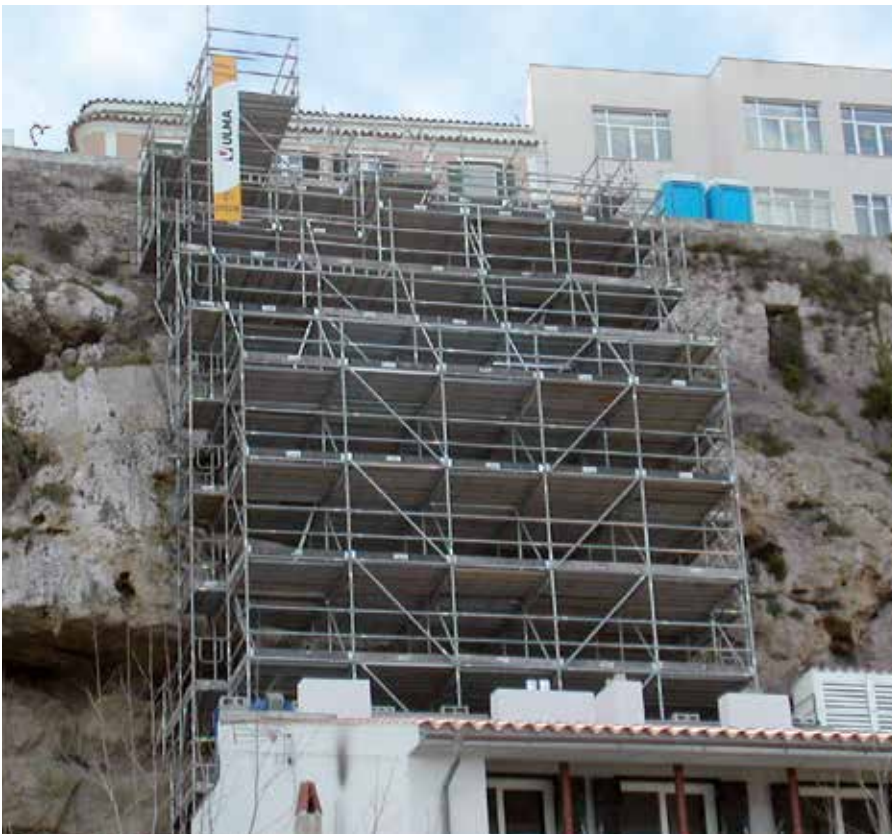
▲ Erection of scaffolding over cliff
