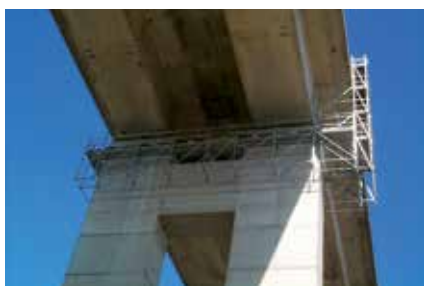
▲ Hanging scaffolding for maintenance works at a viaduct
