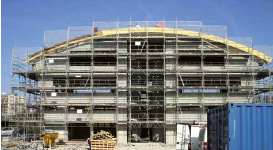
▲ Roof edge protection in new building construction
