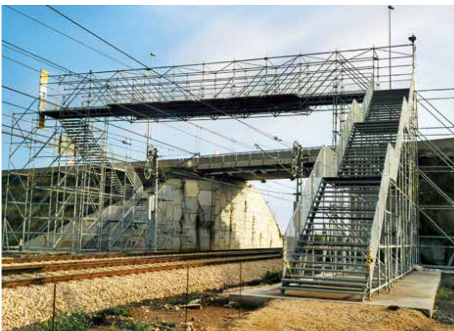
▲ Footbridge to cross over railway line
