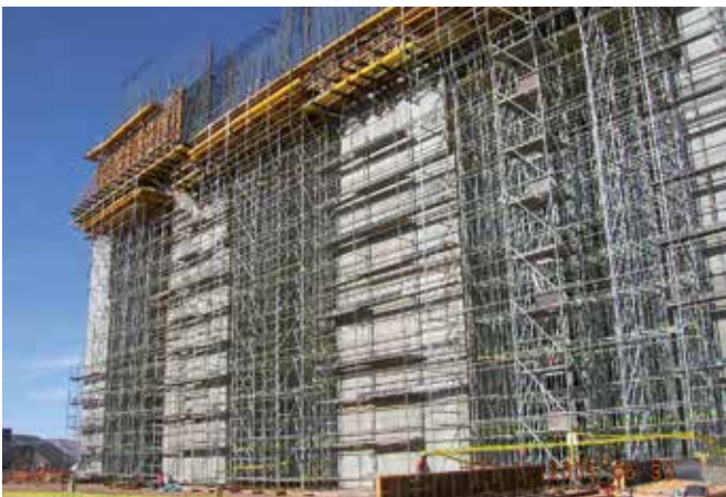
▲ Slab construction at great height
