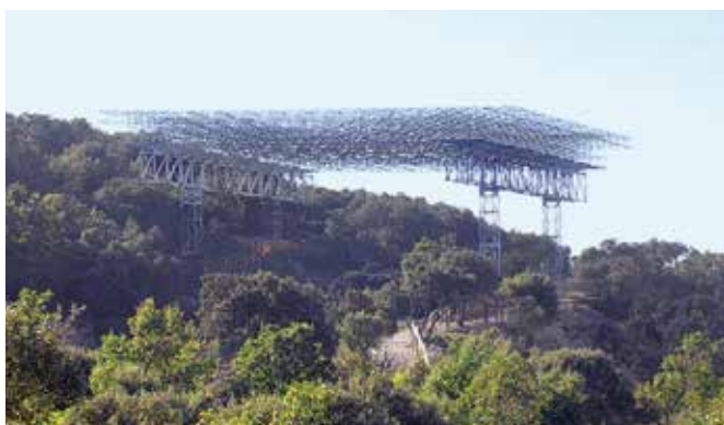
▲ Temporary roof with a span of 22 m erected with standard items of the BRIO Scaffolding system.
