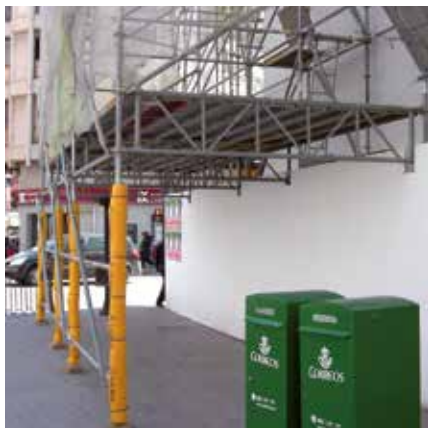
▲ Scaffolding standards secured with protecting tubes in pedestrian walkway
