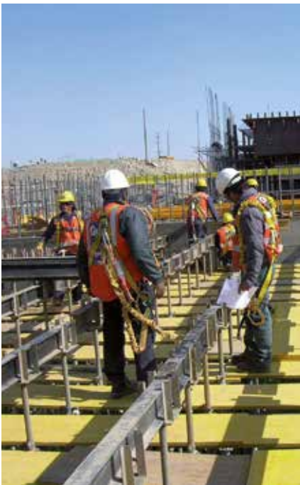
▲ Creation of safe working spaces for formwork erection and at the perimeter ▲
