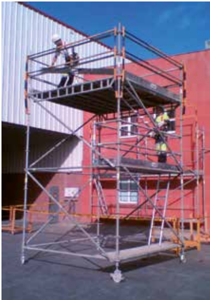
▴ Erection of mobile scaffolding tower with safety guardrail posts.
