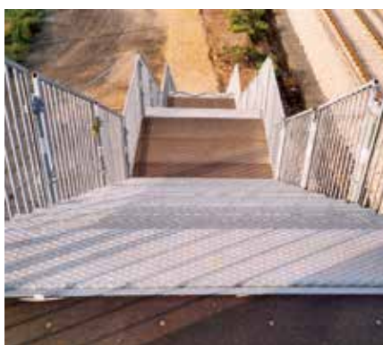
▲ Metal steps and anti-slip wooden stair landing
