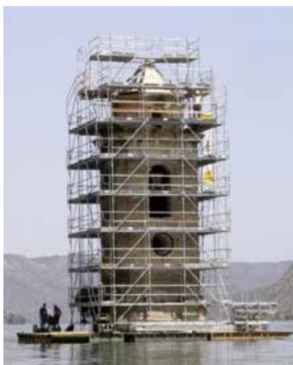
▲ Erection of scaffolding towers
