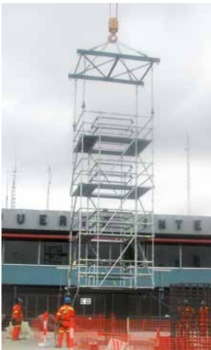
▴ Lifting and moving of towers
