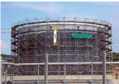
▲ Maintenance of circular tank
