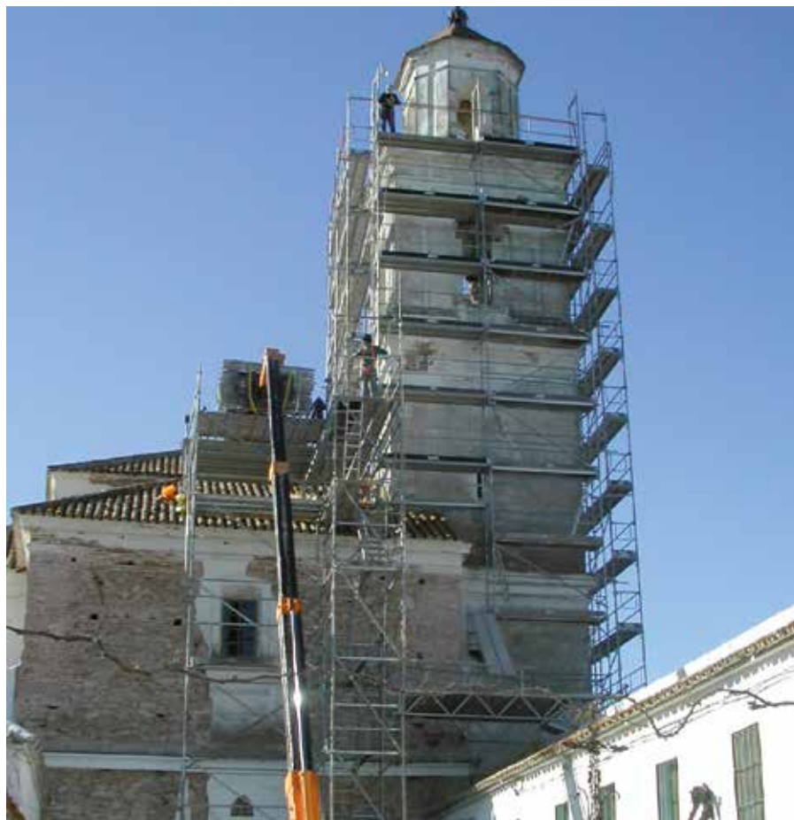
▲ BRIO Modular Scaffolding in the irregular part of the support and DORPA Frame Scaffolding in the upper part ▲
