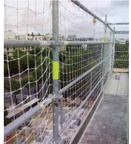
▲ Protection net reinforced at the perimeter
