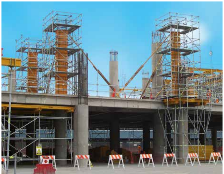
▴ Scaffolding towers for pouring of columns in the extension of the Jorge Chavez Airport, Lima, Peru
