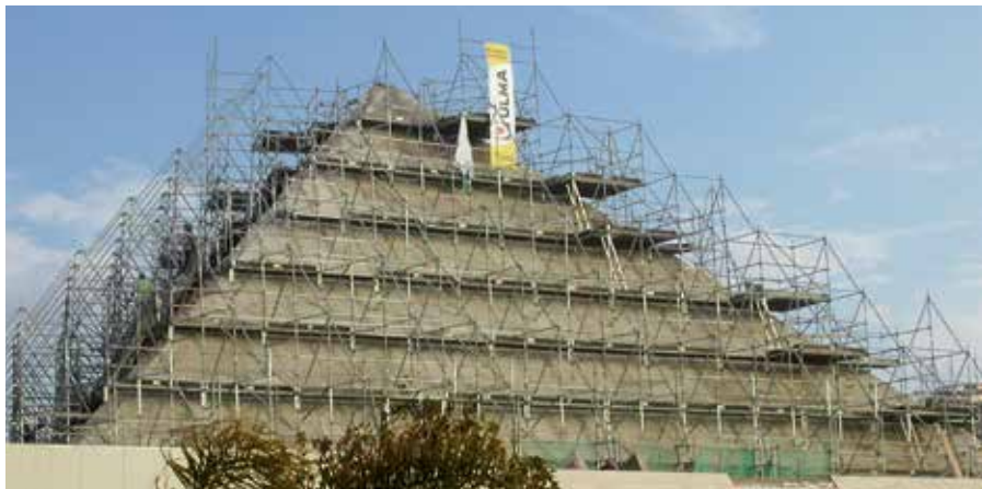
▲ BRIO Modular Scaffolding in inclined façade
