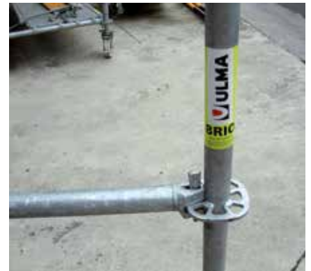
4 Standard and ledger are joined.
