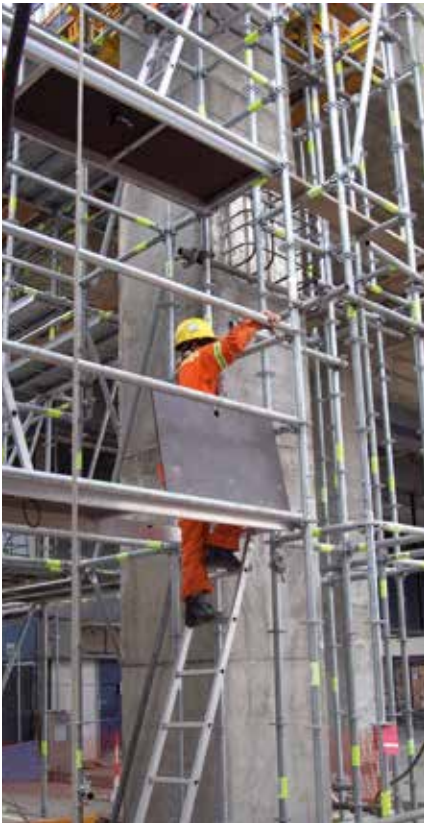
▲ Access via ladder through trapdoor platform
